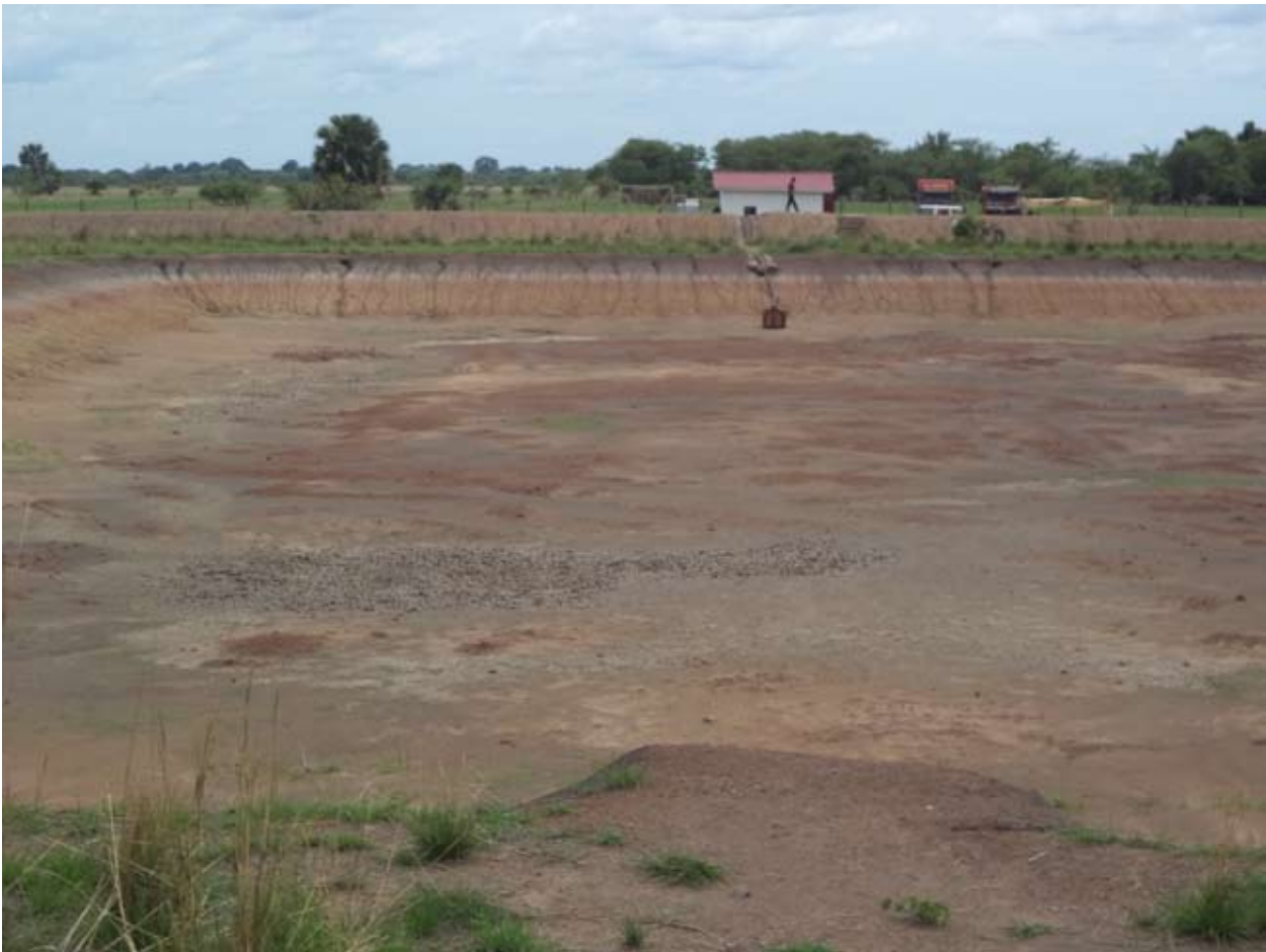
Figure 4. A haffir that never collected water because of inappropriate site selection, at Cieubet, Lake State
