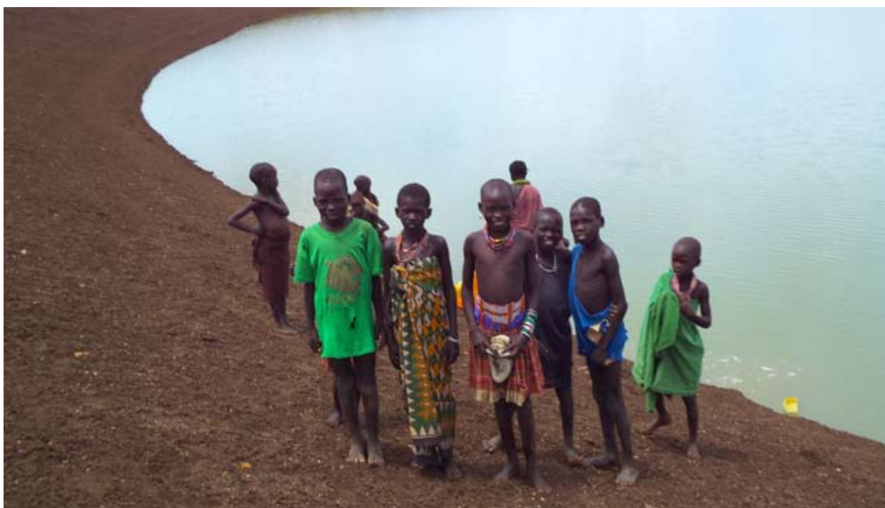
Figure 1. Unprotected water barrier at Nakrumai, Eastern Equatoria State
