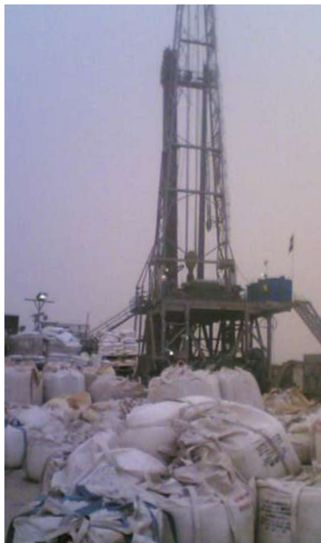
PHOTO 6: Poor storage of chemicals
