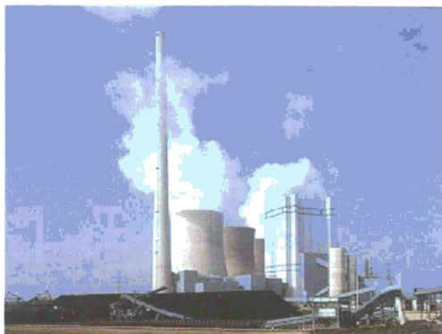
Photo 2.3 Thermal power generation
