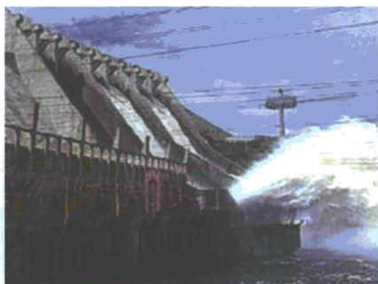
Photo 2.4 Hydro power generation
