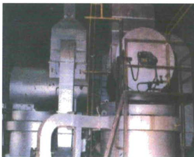
Photo 12.8 Hospital waste incinerator at Safdarjung hospital Source Parivesh Newsletter, Highlights 1998, December 1998, Central Pollution Control Board, Delhi
