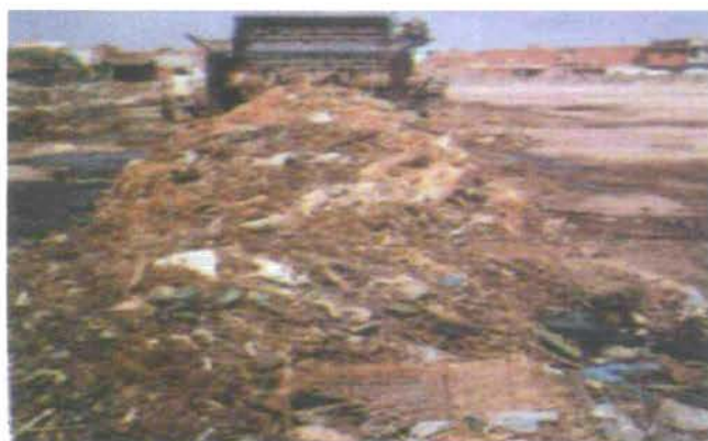
Photo 12.3 Municipal waste being compacted at the dumpsite
