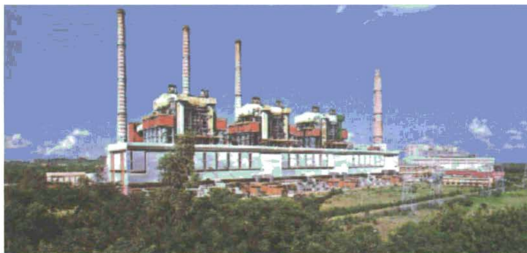
Photo 3.2 Ramagundam super thermal power project
