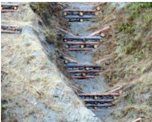
Left: Sketch of the structure of wooden check dams (from Rauch, Rauch and Kirchmeir 2016). Centre and right: Wooden check dams installed in a gully in Jvarboseli village (before and after) ©Deutsche Gesellschaft für Internationale Zusammenarbeit GmbH (GIZ 2019/Sustainable Caucasus)
