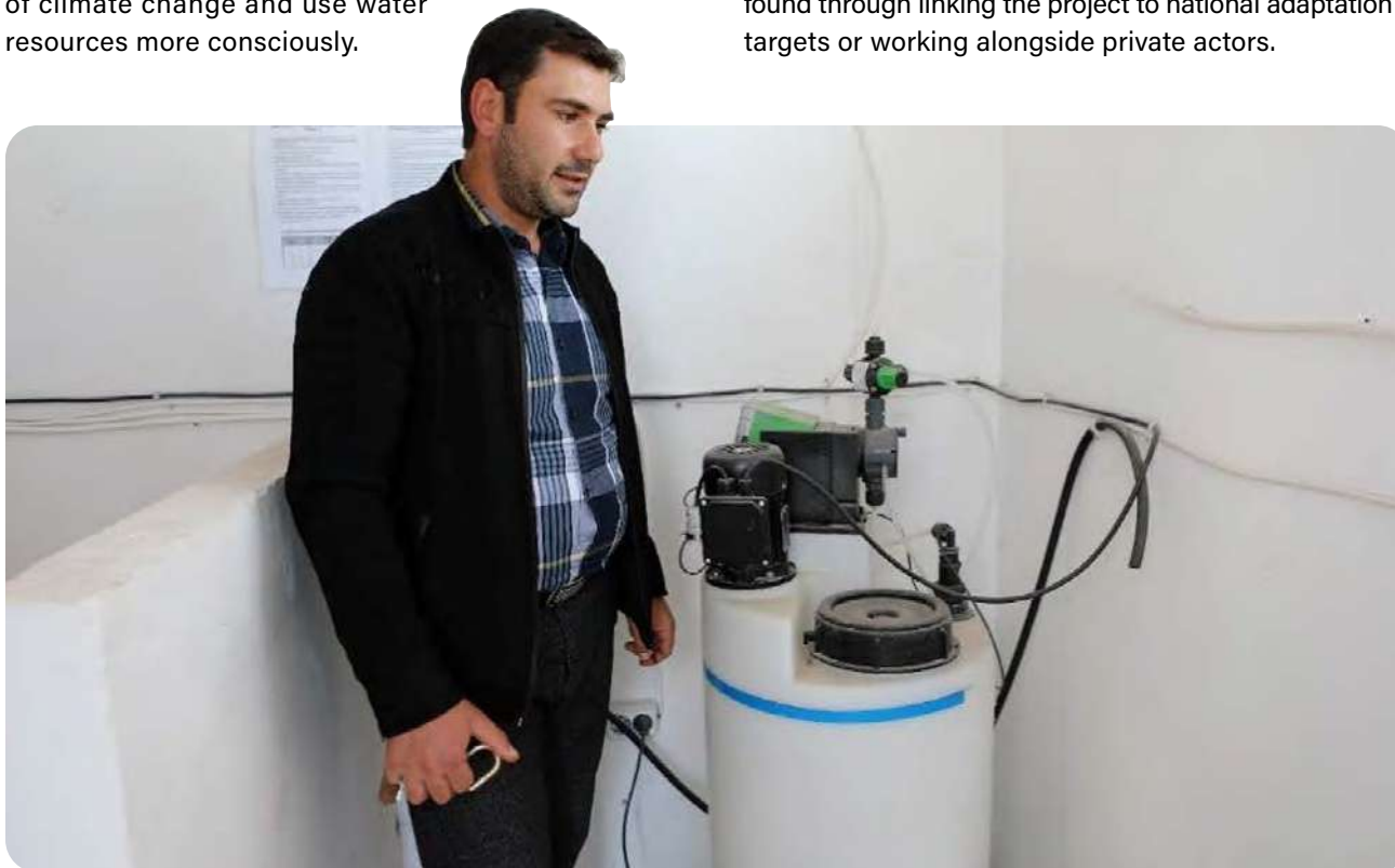
Chlorination station equipment installed in Basen. Hayk Mnatsyan (pictured) is the village administration specialist for the station ©Sustainable Caucasus
