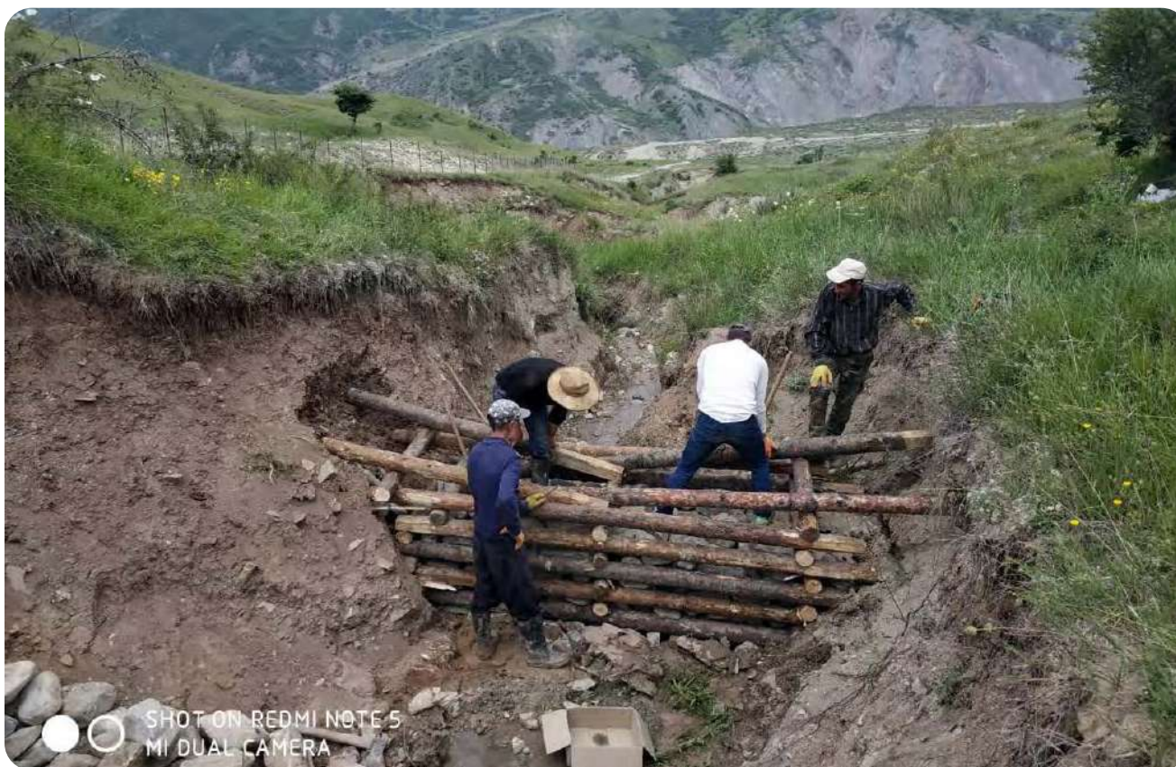
A wooden check dam under construction in the pasture area of the village Ehen, Azerbaijan ©Sustainable Caucasus
