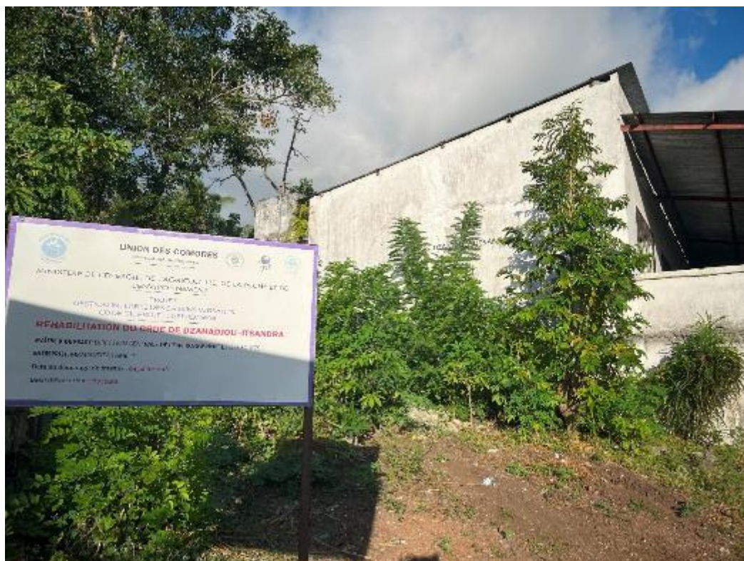
Figure 7: Dzahadjou-Itsandra rehabilitated CRDE (source: Baastel)
