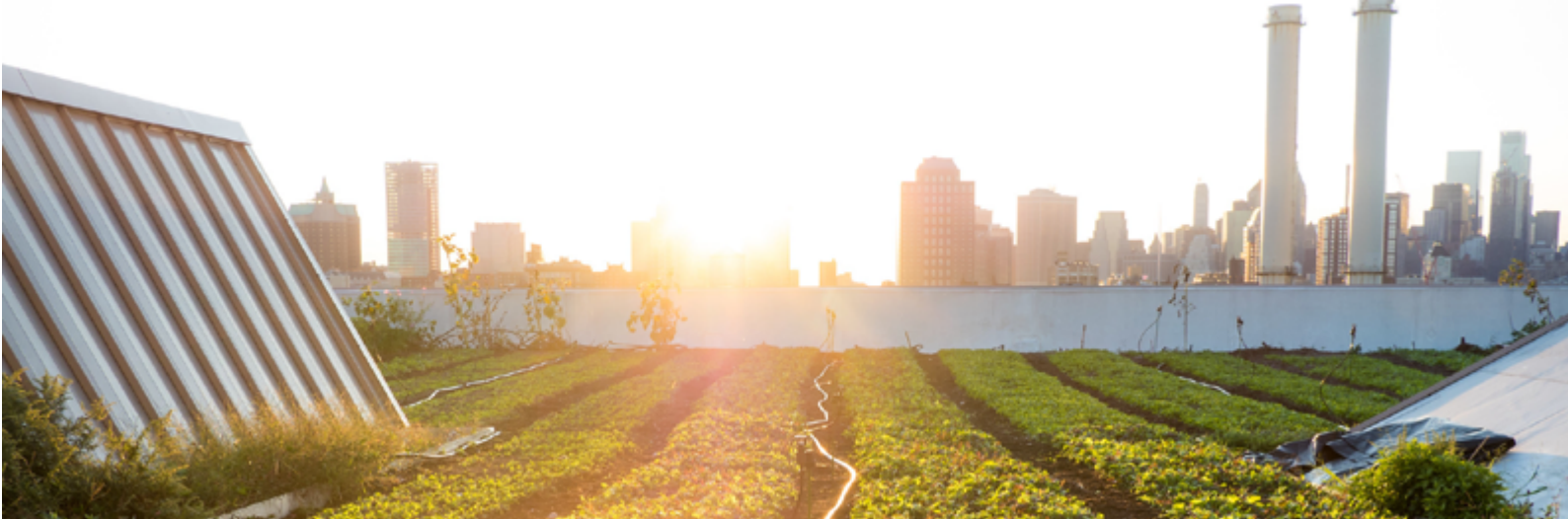
Brooklyn Grange, a rooftop farm in Brooklyn, grows produce atop industrial buildings while demonstrating green-roof benefits such as stormwater retention and urban heat reduction. Photo: Justin. Licence: CC BY 2.0. Flickr.
