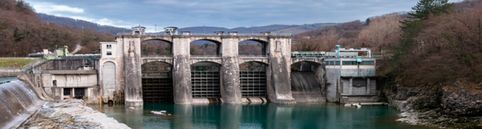
Plave, Slovenia (28 December 2022): The Plave hydroelectric dam on the Soča River, part of Slovenia's renewable power system underpinning its 2050 climate-neutral target. Photo: Taljat. Adobe Stock.
