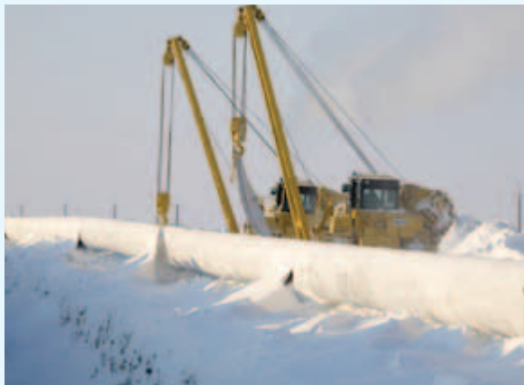
Figure 10.5. Pipeline under construction in the Russian Arctic.
