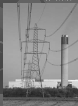
Coal-fired power plant
