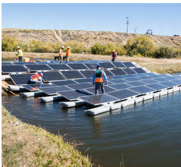
Floating photovoltaics (FPV) Installation in Walden, Colorado (National Renewable Energy Lab)
