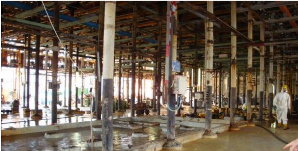
Floor of cell room regularly washed down
