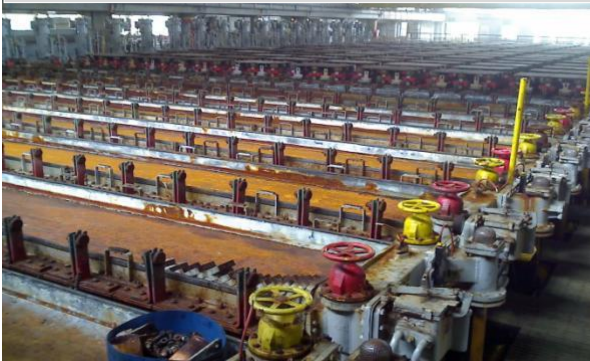
First stage of operations
