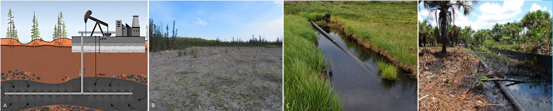
Figure 2 Extraction infrastructure and pipe lines on peatlands: A) scheme of an in-situ oil pad built on peatland (Canada [1]), UNEP 2022 [1]; B) foundation of an oil pad on peatland (Canada), photo: M. Guéné-Nanchen; C) gas pipeline on peatland in Russia, photo: H. Joosten; D) oil infrastructure and contamination in wetland/peatland of the Pastaz-Marañón Basin in Peru, photo [5].
