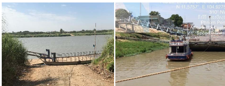
Piers for River Crossing Boat
