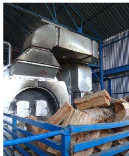
FIGURE 19: Wood drying before use in a boiler fed by woody biomass at Finlays estate (Kericho)
