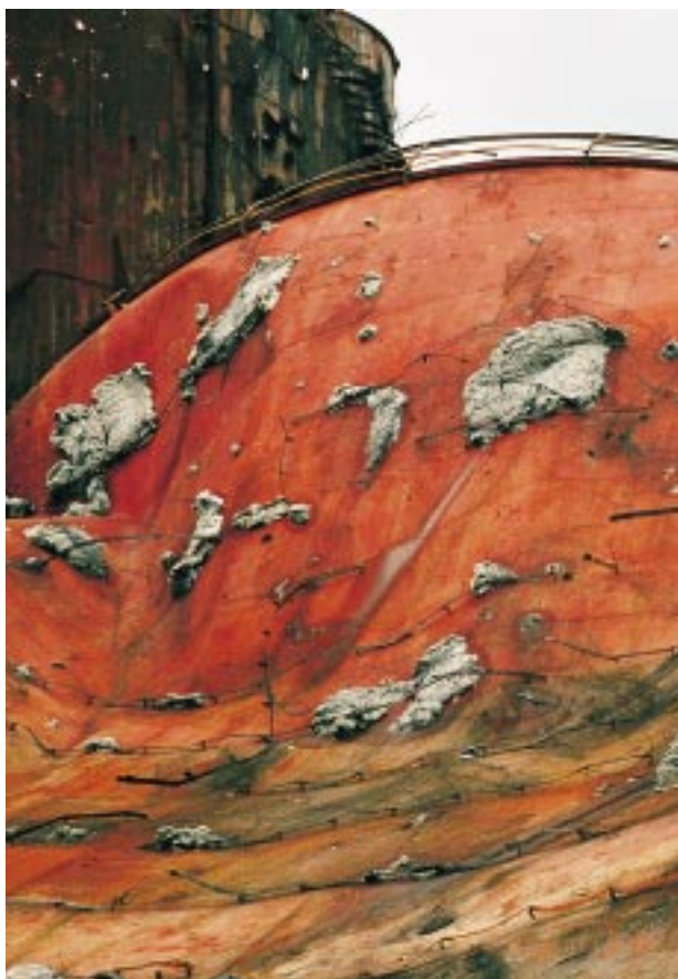
Destroyed oil tank at Novi Sad
