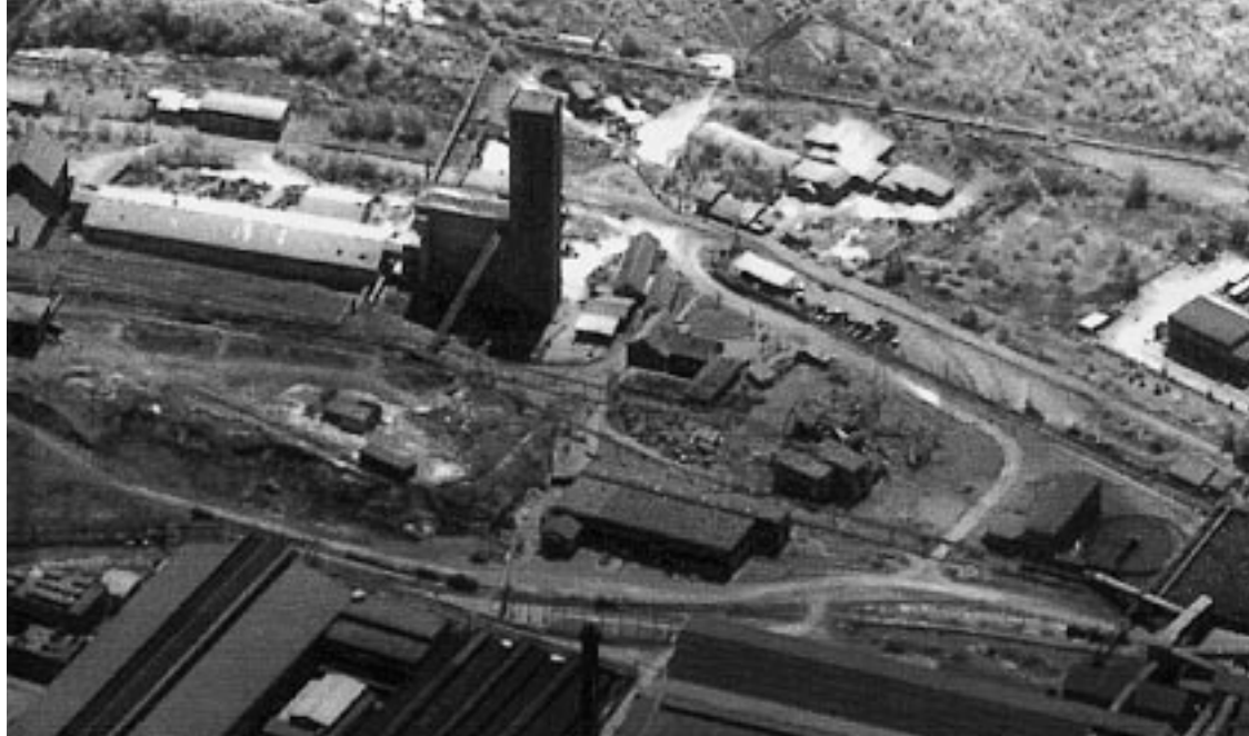
Bor copper smelter and refinery
