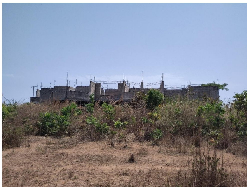
Figure 11: Yundum meteorological headquarters in construction
