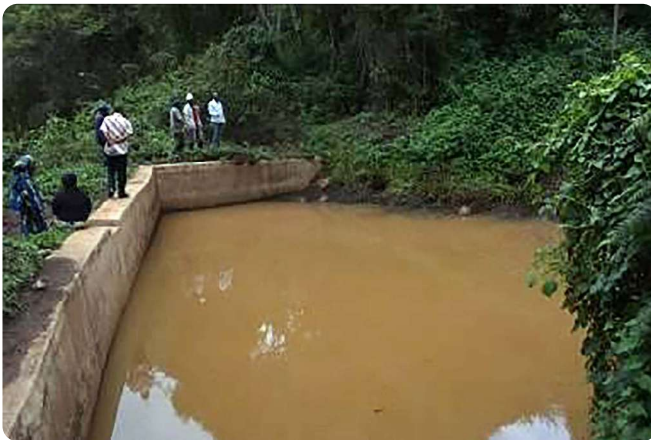
Constructed ndiva supported with concrete ©Hans Komakech
