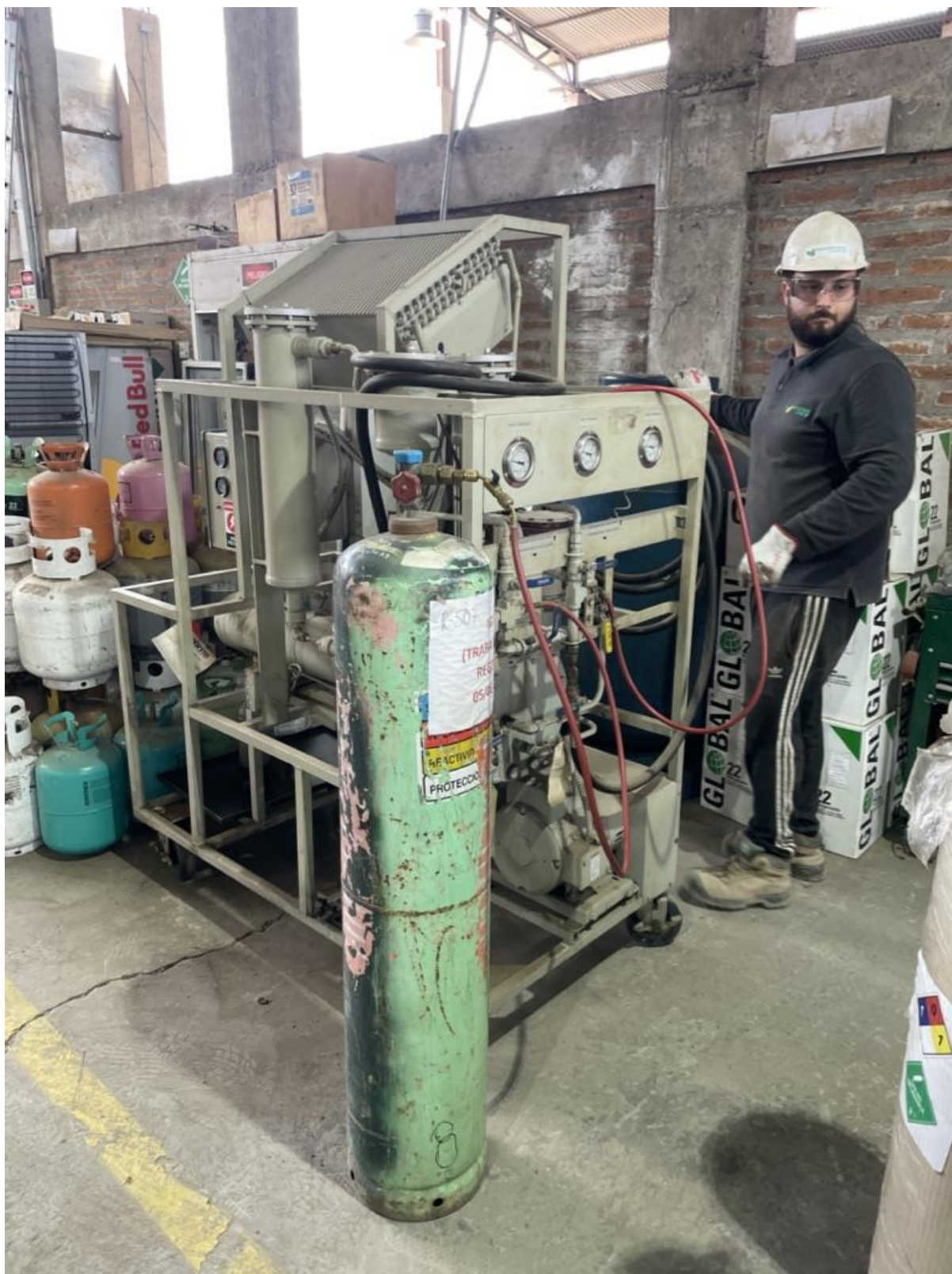
Figure 6 Equipment employed to safely extract and test refrigerant gases from out of use refrigerators in Santiago, Chile, 12/JAN/2023
