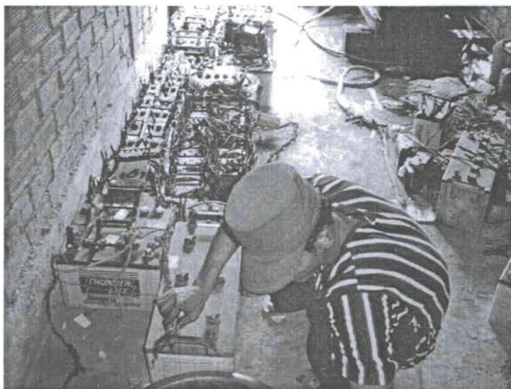
Pic.2.22: LAB recharging service in area close to a bedroom
