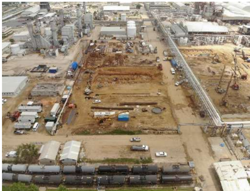
Figure 1. Overhead view of Coatzacoalcos plant construction, September 2021
