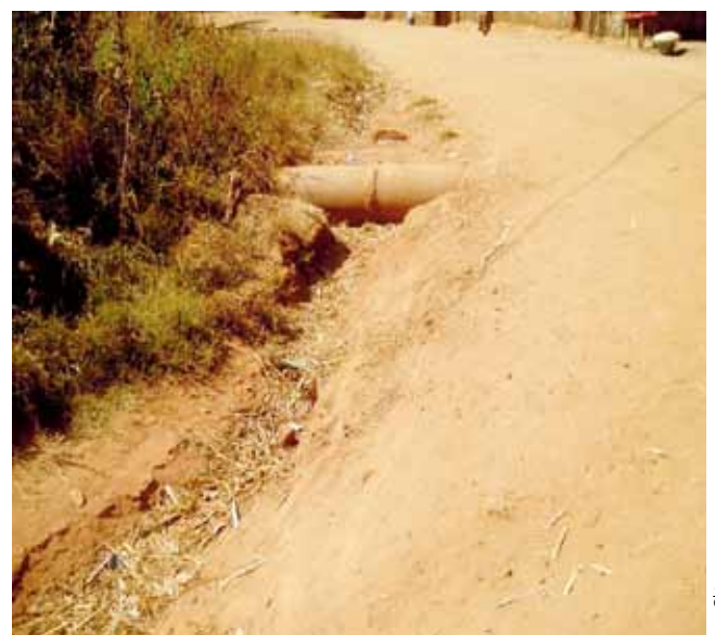
Erosion of road drains.
