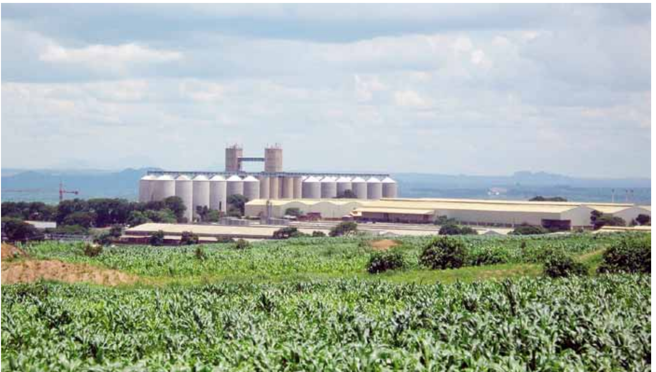
Grain Storage Facility, Photo by Deepa Pullanikattil
