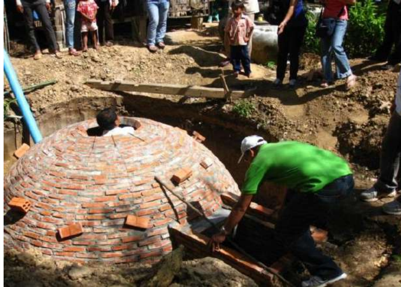
Deployed and constructed 10 Biogas Digesters in Takeo, Cambodia & General Santos, Philippines
