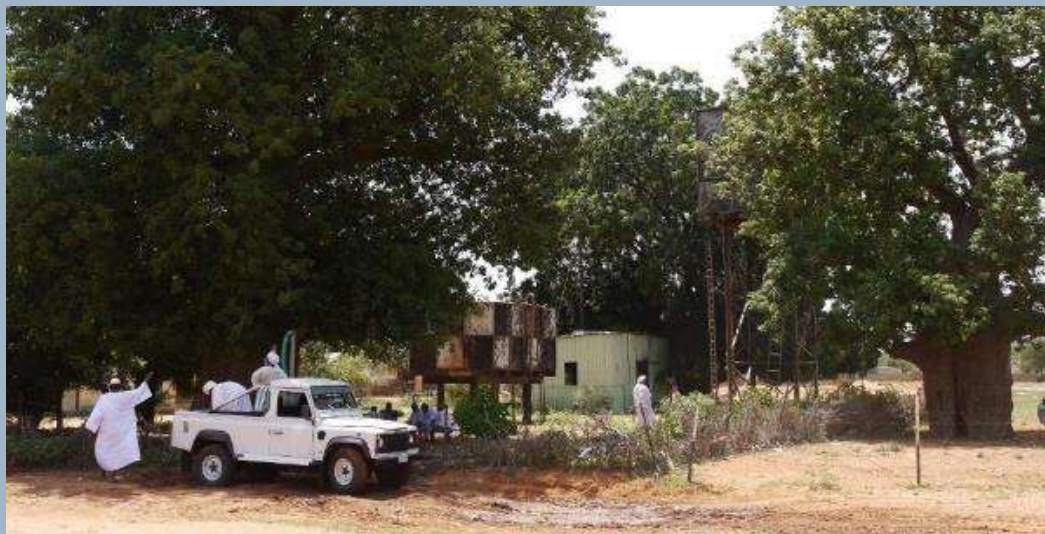
Figure 4.9 The Al Khewei water yard
