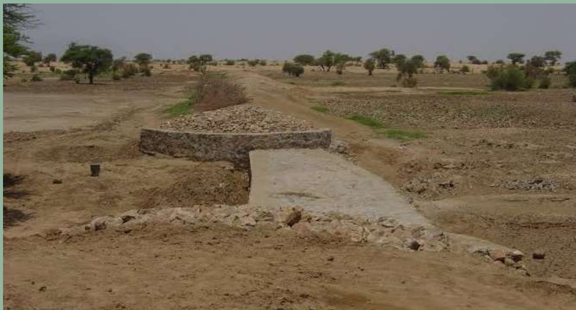
Figure 6.7 A spillway on the water spreading dam in Um Barunga in Darfur. This structure captures a large pool of water on the upstream side (the left in this photo). During the wet season this water can be used to irrigate a crop downstream of the dam. As the flood water recedes, a crop can be grown on the upstream side of the dam (Source: Practical Action)
