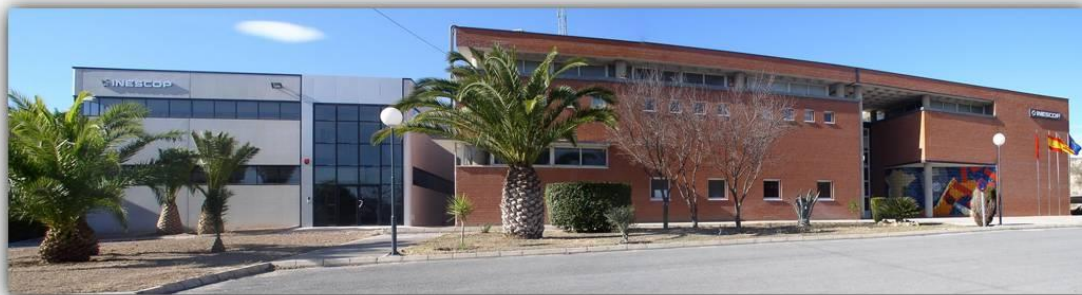
Figure 1. INESCOP's Headquarters in Spain
