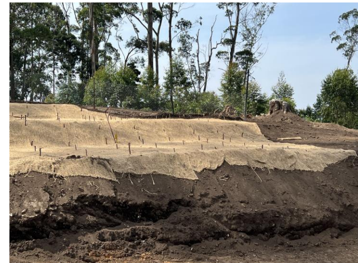
Clean Soil Re-used on-site
