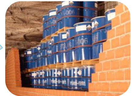
Sealing of by walls
