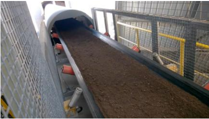
Mercury containing wastes and soils
