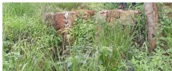
After the project - gully repair
