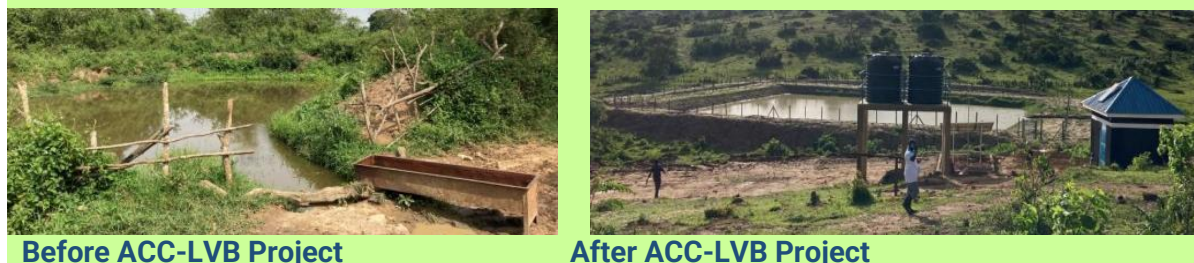
Figure 10: Valley Dam in Mubende, Uganda before (left) and after the project (right)
