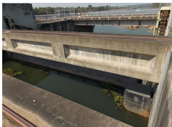
Figure 1 Water gate at Pak Moon Dam
