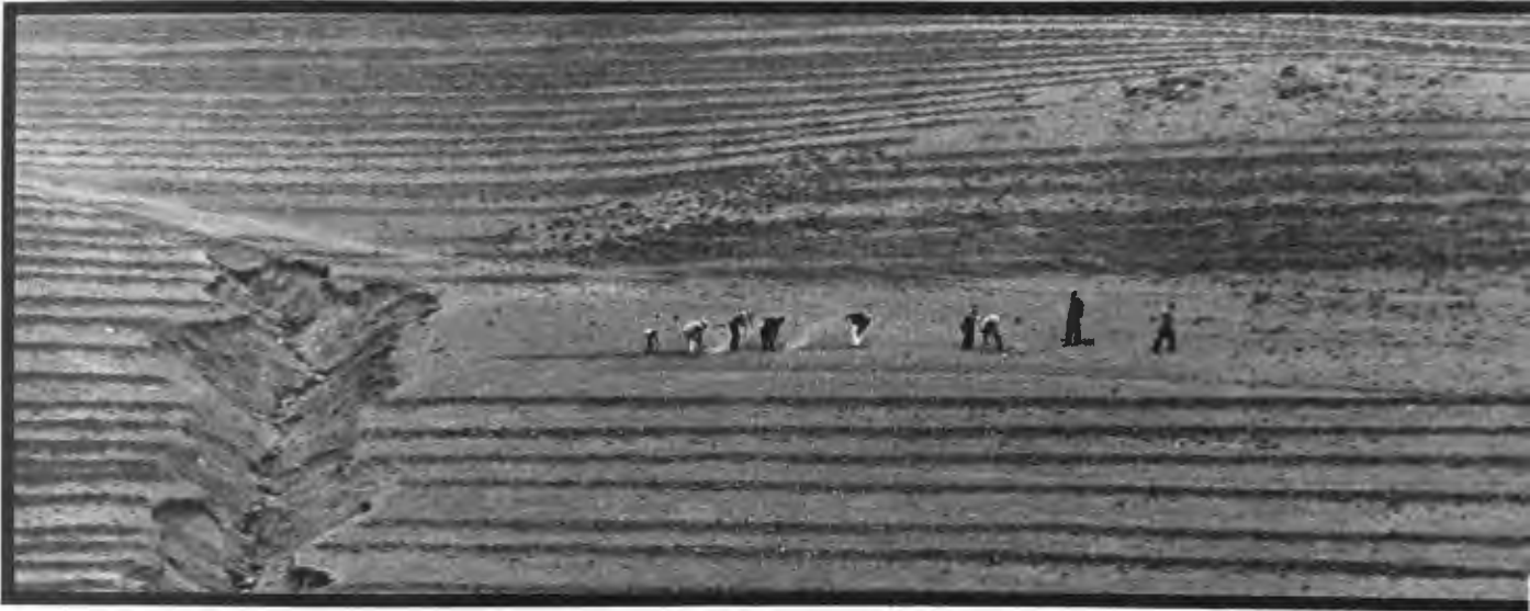
Ditches being dug to prevent soil erosion in Pena Blanca, Chile
