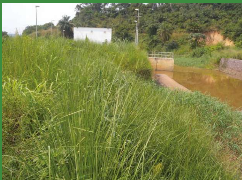
River bank stabilization using vetiver grass. Before (top) and after (bottom) intervention at intake point of the REGIDESO water treatment plant.
