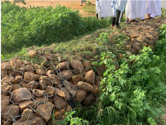
Figure 8: Bank stabilization (Ndoumally)
