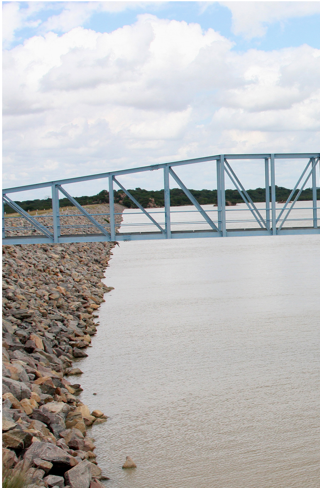
Letsibogo dam Photo credit: Photography Section, BOPA
