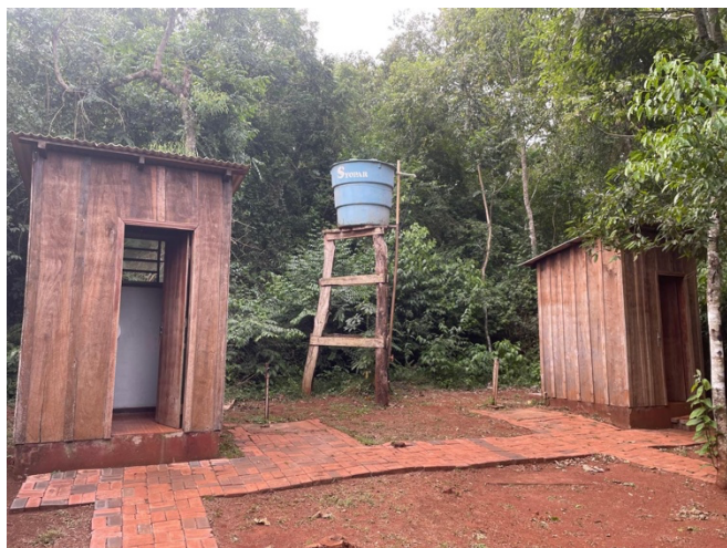
Water infrastructure installed by the project resulted in water access to toilets that were previously not used because of lack of water
