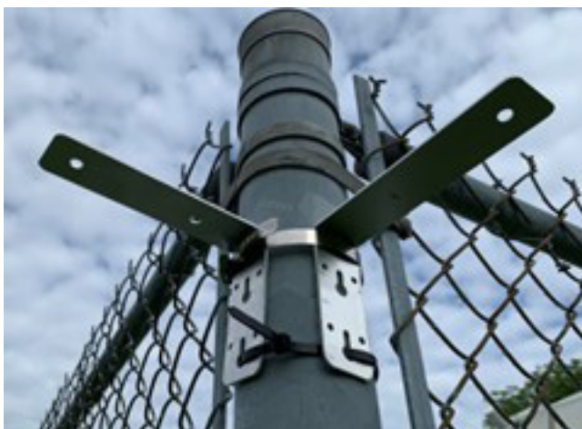
Figure 3. Visualization of mounting brackets for installing MerPAS® samplers
