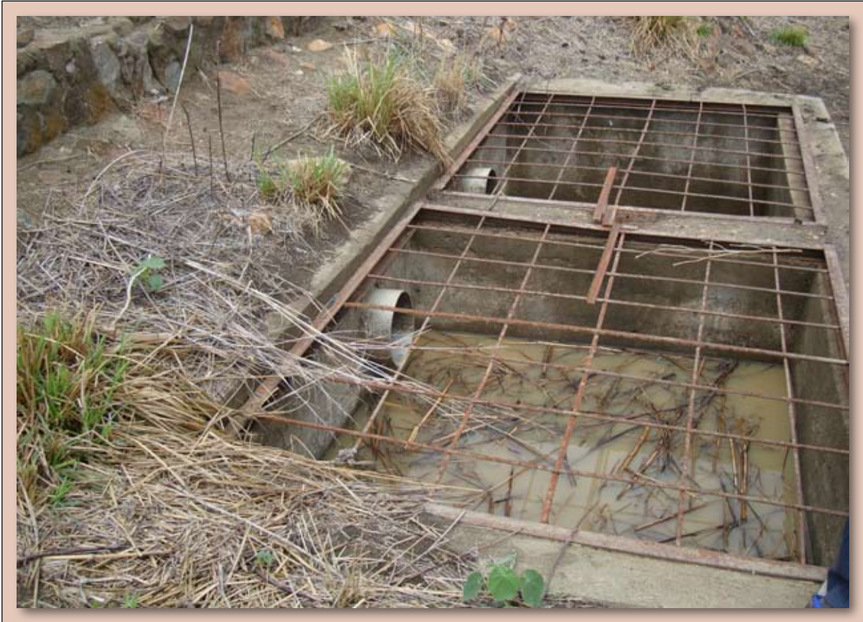
Figure 7. Properly sized inlet box and inlet pipes (Lokoges haffir , Kapoeta North County, Eastern Equatoria)
