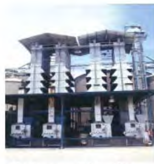
Drying ovens in Costa Rica
