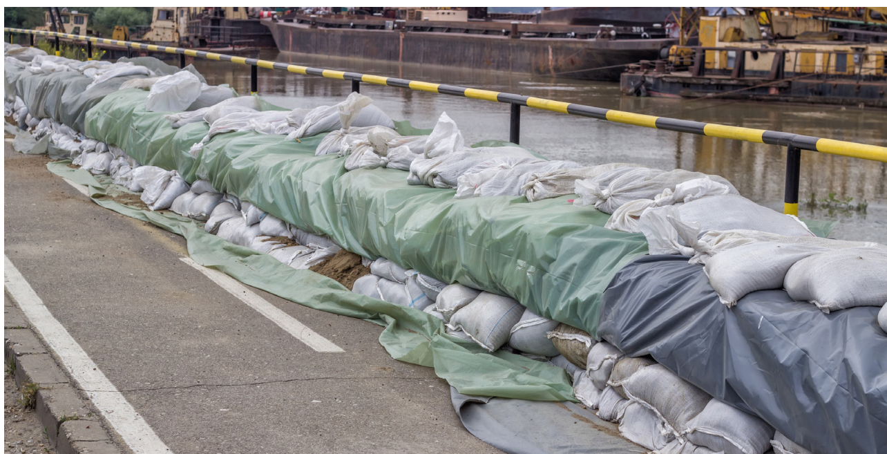
Wall of sandbags for flood defense, sandbag barricaded Photo: iStock
