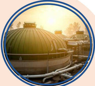
Generate green energy
