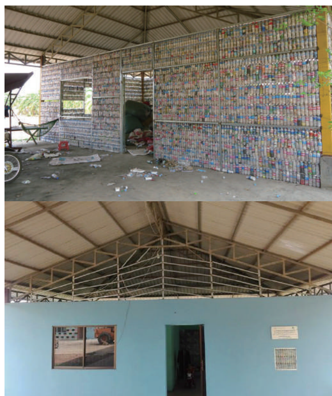
Figure 8: Use of Plastic Bottle Bricks for Construction at the Composting Centre
