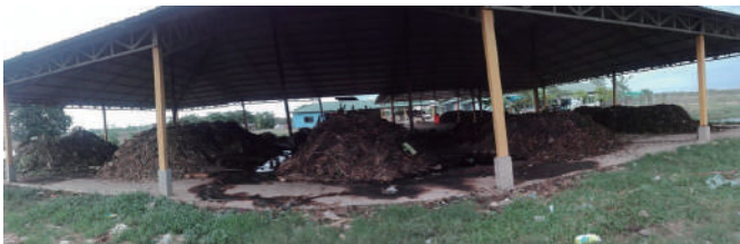
Figure 7: Composting Plant Operated by COMPED
