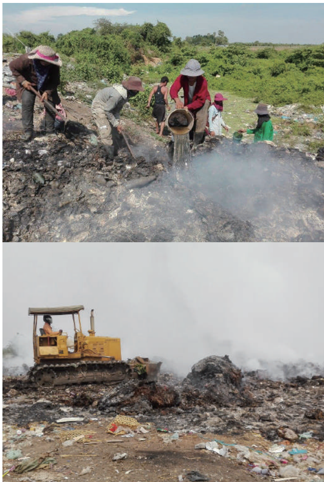
Figure 13: Extinguishing Landfill Fire using Water and Soil
